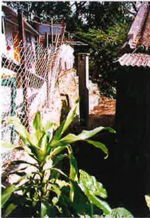
7SE-A/R102 OVERALL VIEW
