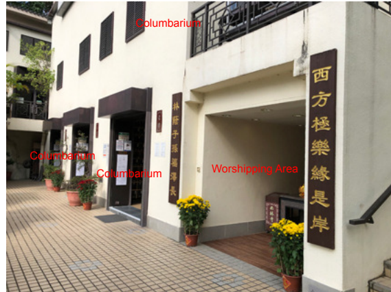
Photo 5: Building D (G/F & 1/F)
